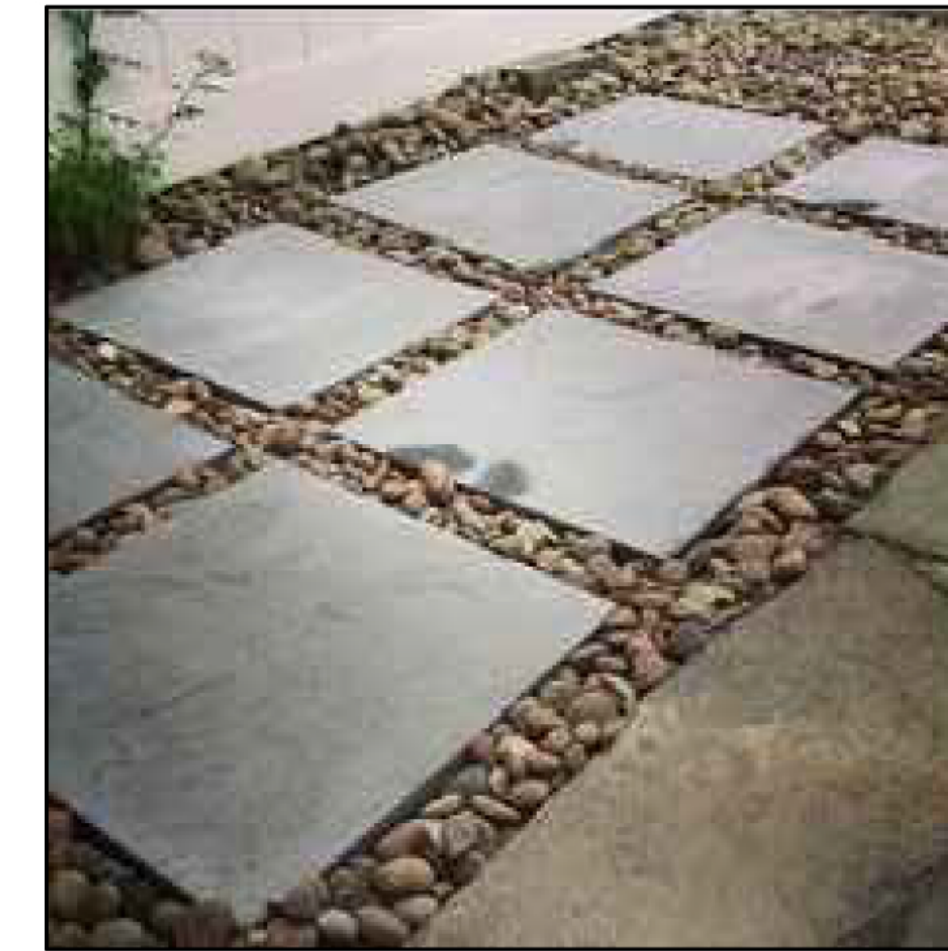
PEBBLES INBETWEEN THE PAVEMENT BLOCKS
